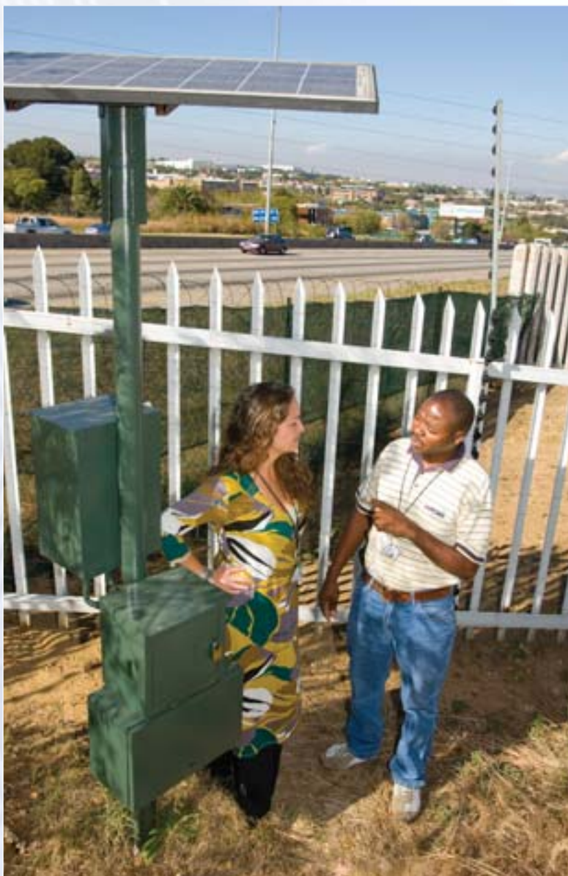
Ronel Eksteen, Bytes Business Park facilities manager and Kleinbooï Mashiyé, assistant, at the solar powered security fence at Bytes Business Park.
