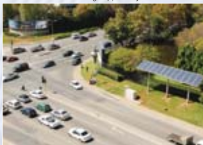
Solar powered traffic lights at intersections in Johannesburg supplied by Rentech.
