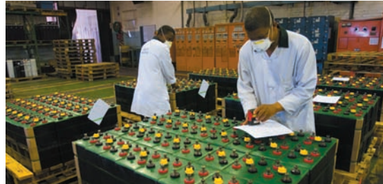
Final inspection of industrial battery cells by Quality Department – Port Elizabeth Factory, before being booked into stock and despatched to Ophirton DC Power Marketing warehouse.
