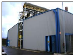
Above and below: Typical installation of a 3MVA Jenbacher gas-engine installation in co-generation applications
