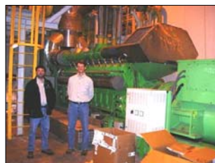
Above and below: Typical installation of a 3MVA Jenbacher gas-engine installation in co-generation applications
